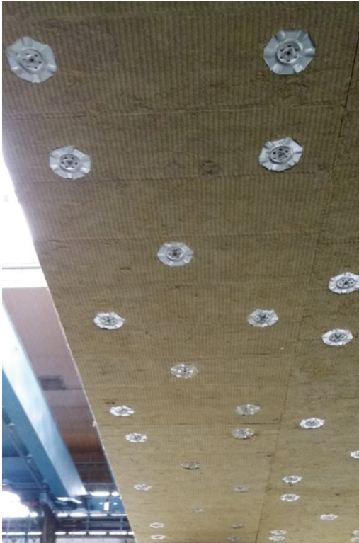
Fire protected concrete slab.
