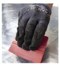
Duct flanges or suspensions are integrated into the insulation. Cut the incisions as accurately as possible so that the air gaps are not too large.
