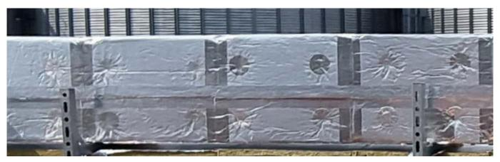
To seal the welding pins, use the PAROC® Clad Alu Dots. To increase the tightness of the PAROC® Clad Alu Dots, a plastic spatula is also recommended as a support. A cardboard template can be produced to optimise the appearance of the welding pins.
