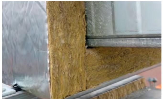
The two sides of the duct (*a*) are cut to size including the insulation thickness ( $2xs$ ).
