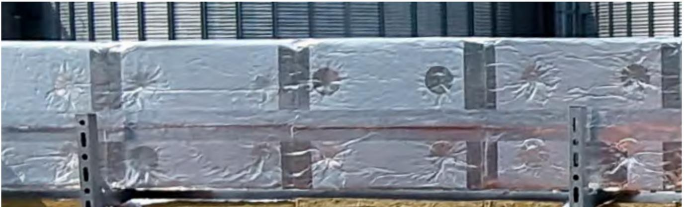
To seal the welding pins, use the PAROC® Clad Dots. To increase the tightness of the PAROC® Clad Dots, a plastic spatula is also recommended as a support. A cardboard template can be produced to optimise the appearance of the welding pins.
