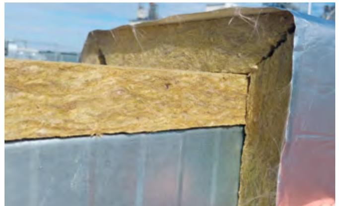
After the second half has been produced, the slabs and V-cuts are fixed with spray adhesive and secured with welding pins (Option 1), then all joints are taped with PAROC® Clad Alu Tape or PAROC® Clad Tape.
