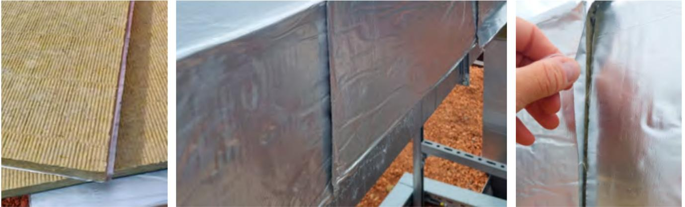
All longitudinal and butt joints are glued or sealed with PAROC® Clad Alu Tape or PAROC® Clad Tape. A plastic spatula is recommended for evenly pressing the PAROC® Clad Alu Tape or PAROC® Clad Tape onto the slabs to ensure a permanently tight bond.
