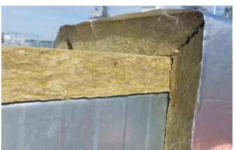
After the second half has been produced, the slabs and V-cuts are fixed with spray adhesive and secured with welding pins (Option 1), then all joints are taped with PAROC® Clad Alu Tape.
