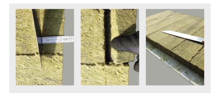
Mount the PAROC® Pro Lamella Mat Clad on the duct sides and back. In order to make the installation easier, a spray adhesive could be used. For the permanent mechanical fixation on the duct we recommend using welding pins; with a maximum distance of 300 mm. To ensure a uniform positioning of welding pins, we recommend using a corresponding template.
