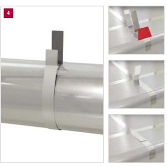
**4.** For permanent **waterproofing**, apply PAROC Clad Tape or PAROC Clad Alu Tape to all **connecting joints** and **lengthwise seams**.
