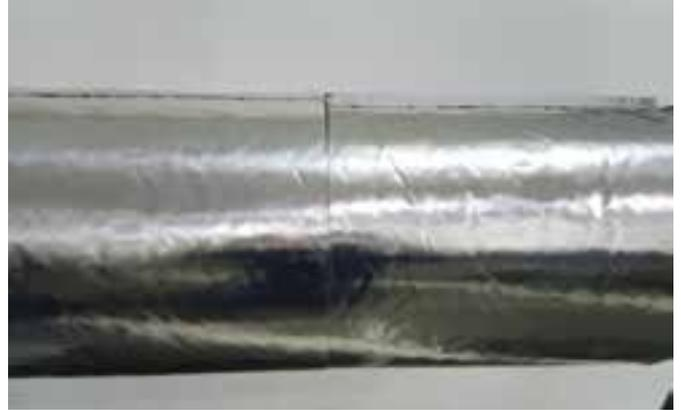
With small pipeline diameters, high circumferential stresses may occur. To ensure that the mat is tightly pulled together, an PAROC Clad Tape with the sealing and adhesive compound is applied around the circumference (2 times) to secure the mat firmly on the folding. Then the tape is also glued on the longitudinal folding;
