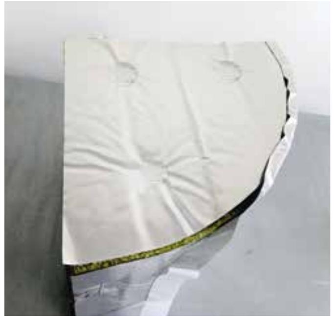
All points of welded pins must be secured with PAROC Clad Dots. The fold points of individual mats are taped as follows:
