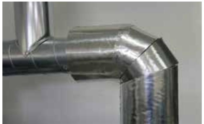
Place the cut out elements are put on the elbow and cover the circumference joints with PAROC Clad Tape with the sealing compound.
