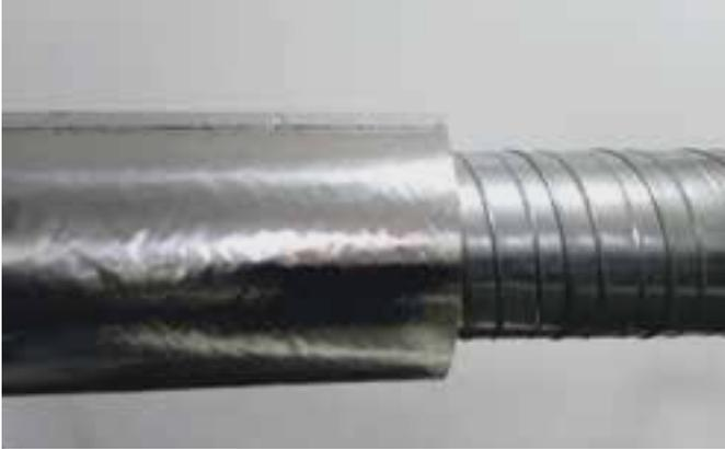
The calculated length of the mat should be cut along the folding lines of the lamellas. The folding lines (strips) of the lamellas help us to cut the mat straight to its edge. Cutting in the other direction will make it impossible to wrap the mat around the pipeline;
