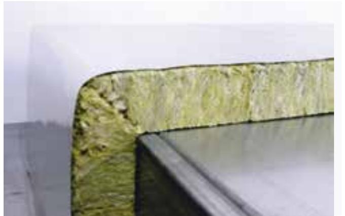
A different way is presented below. The fold points are cut at a 45° angle with consideration of two thicknesses of the applied insulation material. This cut can be made with a cutting strip with the same angle. The fold points are cut to make the mat edges easier to fold.
