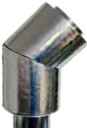
3. The cut out elements should be placed on the bend - the elbows below 90° - and the longitudinal and circumferential joints should then be covered with PAROC® Clad Tape or PAROC® Clad Alu Tape.
