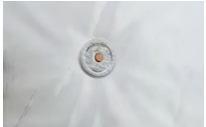
All folds of the individual mats and the points of welded pins should be secured with PAROC® Clad Dots. We recommend that you use a spatula to ensure that the dots adhere tightly to the lining. The length of the pins should fit the insulation thickness.
