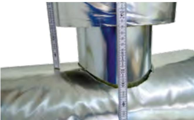
1. First, insulate the section of the pipeline to which the tee connects; Then, measure the tee:
