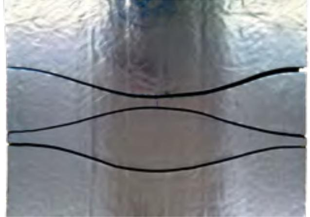
**7.** Any cut to fit sections must be secured by minimum 2 aluminum bands and tape according to the description above.
