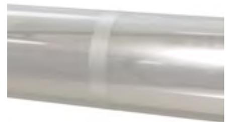
**4.** Always make sure that tape is applied without wrinkles and openings. Use a spatula to smoothen out any air bubbles. There must be no gaps or "pockets" where water can accumulate.
