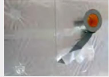
**Seal all open edges with PAROC® Clad Tape or PAROC® Clad Alu Tape; use PAROC® Clad Dots for the welding pins.**
