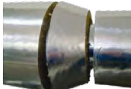
**5.** Seal the transverse joints with PAROC® Clad Tape or PAROC® Clad Alu Tape.
