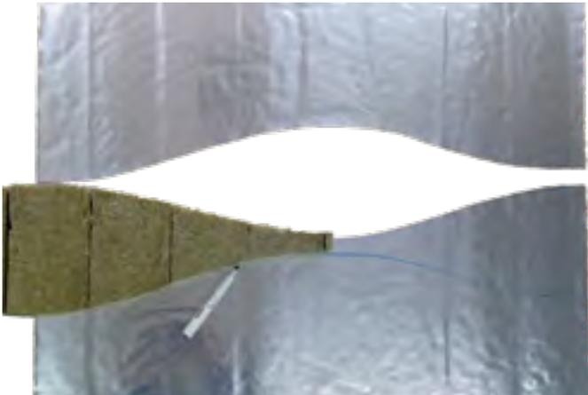
**8.** Place the cut out elements are put on the elbow and cover the circumference joints with PAROC® Clad Tape or PAROC® Clad Alu Tape.
