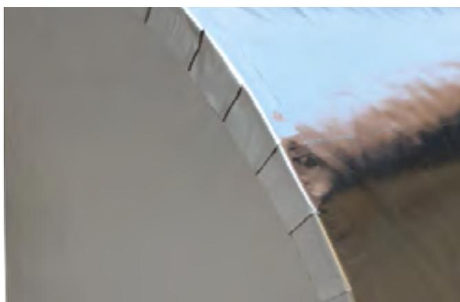
Possible air pockets under the PAROC® Clad Tape or PAROC® Clad Alu Tape should absolutely be avoided. Therefore, post-processing is done using a spatula.
