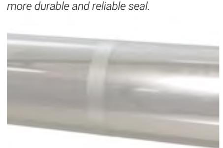
**4.** Always make sure that tape is applied without wrinkles and openings. Use a spatula to smoothen out any air bubbles. There must be no gaps or "pockets" where water can accumulate.
