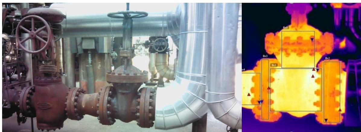
*Insulating one DN 300 valve with a surface temperature of 150 °C and operating all year can save annually 15 MWh and 3 t of CO<sub>2</sub> eq. emissions. Calculated with an energy price of 20 €/MWh this saves 300 € per year. The insulation investment offers a payback time of less than two years.*
