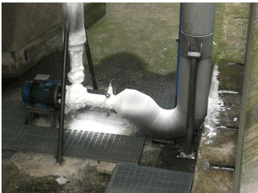
*Pump fully covered with ice breaks down*
