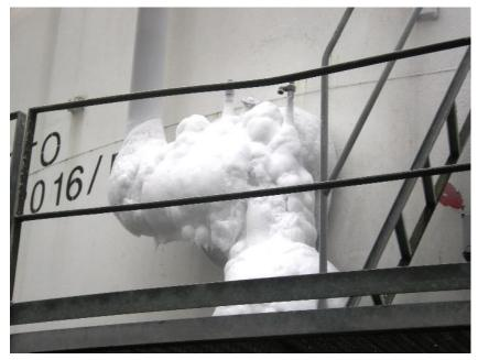
Valve fully covered with ice can no longer be operated
