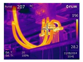
Uninsulated lines with a surface temperature above 200 °C were identified during the TIPCHECK.
