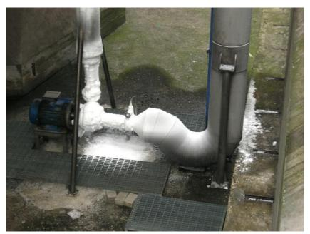
Pump fully covered with ice breaks down
