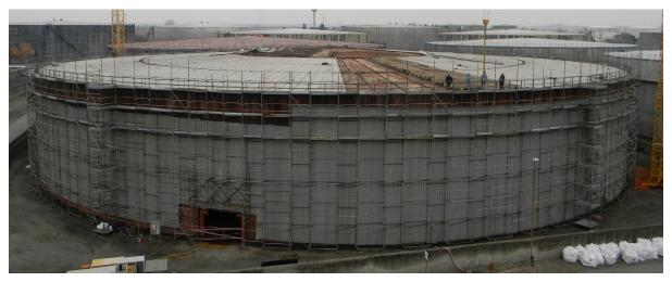
BEFORE: An aged oil storage tank in a refinery had a heavily corroded roof and urgently needed repair
