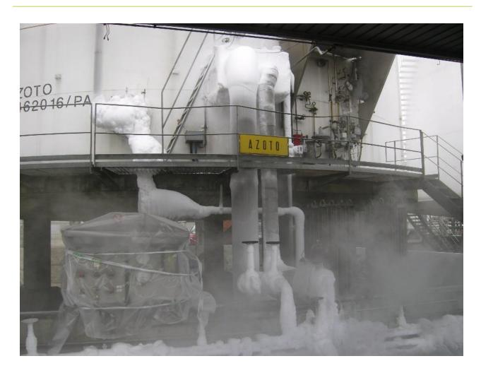
Control panel "protected" with plastic sheeting from the dripping condensation water. Extensive ice formation on pipes and valves
