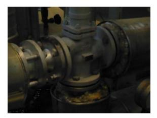
Thermographic inspections identify dangerously high surface temperatures on insulated and uninsulated equipment like on this uninsulated valve and the connected flanges.
