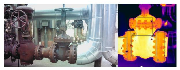
Insulating one DN 300 valve with a surface temperature of 150 °C and operating all year can save annually 15 MWh and 3 t of CO₂ eq. emissions Calculated with an energy price of 20 €/MWh this saves 300 € per year. The insulation investment offers a payback time of less than two years.
