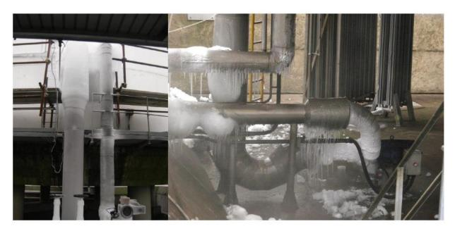
Broken vapour barriers and insufficient insulation caused ice to form around these pipes causing both process control and structural problems
