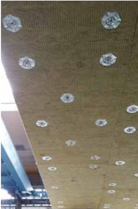
Fire protected concrete slab.
