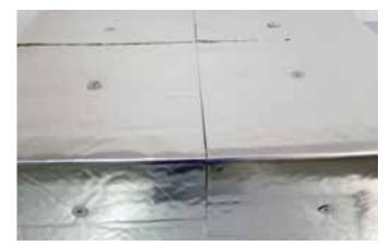
All folds of the individual mats and the points of welded pins must be secured with PAROC Clad Dots. We recommend that you use the spatula to ensure that the dots adhere tightly to the lining.
