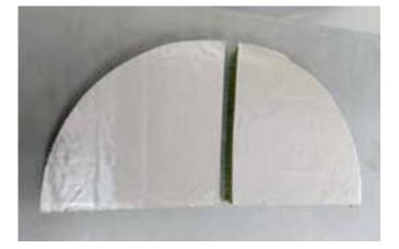
Cut out two (mirror) arc elements for the side surfaces of the elbow and a segment for the arc surface of the elbow;
