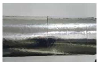
With small pipeline diameters, high circumferential stresses may occur. To ensure that the mat is tightly pulled together, an PAROC Clad Tape with the sealing and adhesive compound is applied around the circumference (2 times) to secure the mat firmly on the folding. Then the tape is also glued on the longitudinal folding;
