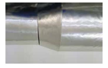
Seal the transverse joints with PAROC Clad Tape with the sealing compound.
