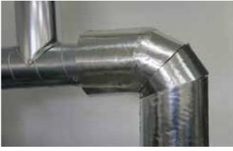
Place the cut out elements are put on the elbow and cover the circumference joints with PAROC Clad Tape with the sealing compound.
