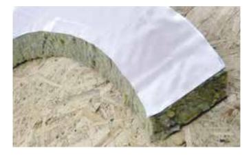
Cut out the mat element at a slanting angle so that after cutting out it may complete the insulation at the reduction spot;
