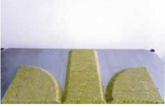
Cut the sections intended for the elbow sides and the arc surface of the elbow at a 45° angle in order to avoid having to tape up the entire insulation thickness;
