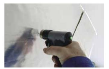
the mat is installed to the duct by placing it on the duct surface and matching the cuts to the edges while simultaneously piercing the lining with the pins and welding them to the duct surface.
