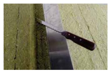
A different way is presented below. The fold points are cut at a 45° angle with consideration of two thicknesses of the applied insulation material. This cut can be made with a cutting strip with the same angle. The fold points are cut to make the mat edges easier to fold.
